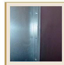
5/16" bolts with serrated lock nut
