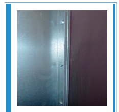
5/16" bolts with serrated lock nut
