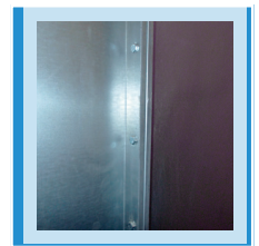
5/16" bolts with serrated lock nut
