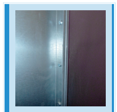
5/16" bolts with serrated lock nut
